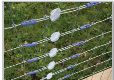
Join horse mesh using Gripple Plus and Twisters
