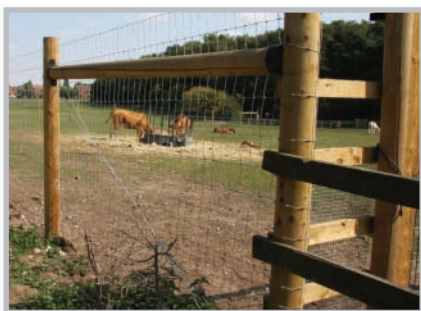
Brace H-Posts with a Gripple Plus Anchoring Kit (GPAK)
