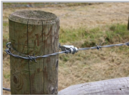
Terminate barbed wire using a Gripple T-Clip 2
