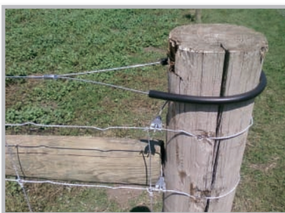
Terminate electric fencing with Gripple Plus and insulation tubing
