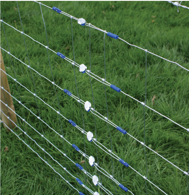
Stock fence repair using Gripple Plus Medium.
